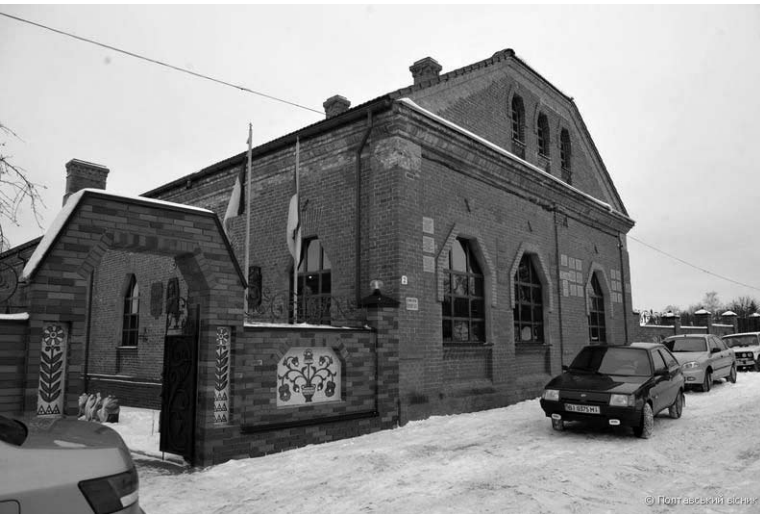
The Krychevsky Museum, building designed by V.H.Krychevsky
